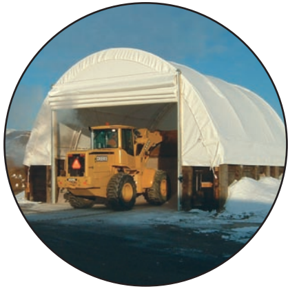
32' x 32' Ponywall Diamond Shelter used by Department of Highways for salt storage.
